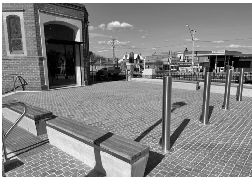
Photo 6: New main entrance
